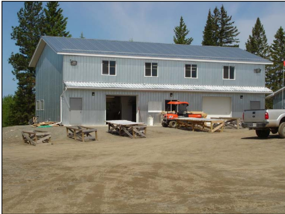
Plate 1 – Rainy River Gold Project (RRGP) core processing facility
