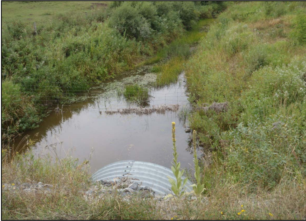
Plate 29 – Pinewood River upstream location culvert crossing (August 2011)
