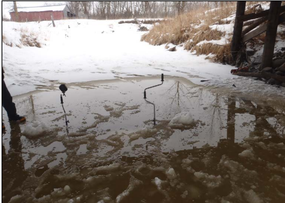
Plate 32 – Immediately downstream of Water Survey Canada Station (05PC023) at Pinewood River bridge, Highway 617
