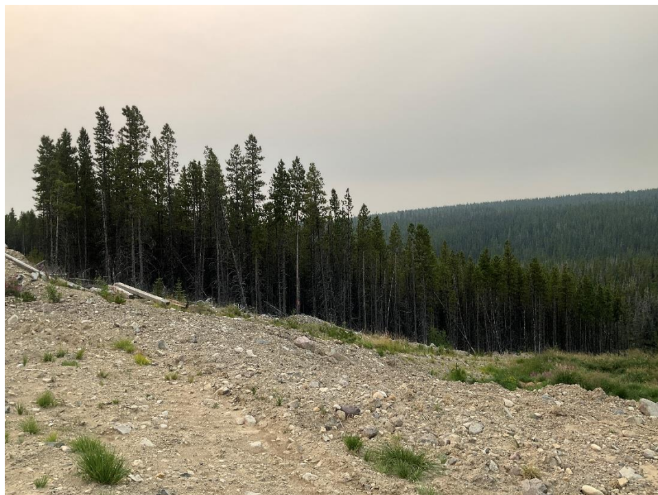
Photo 6. Work area surveyed near septic field August 22, 2023.
