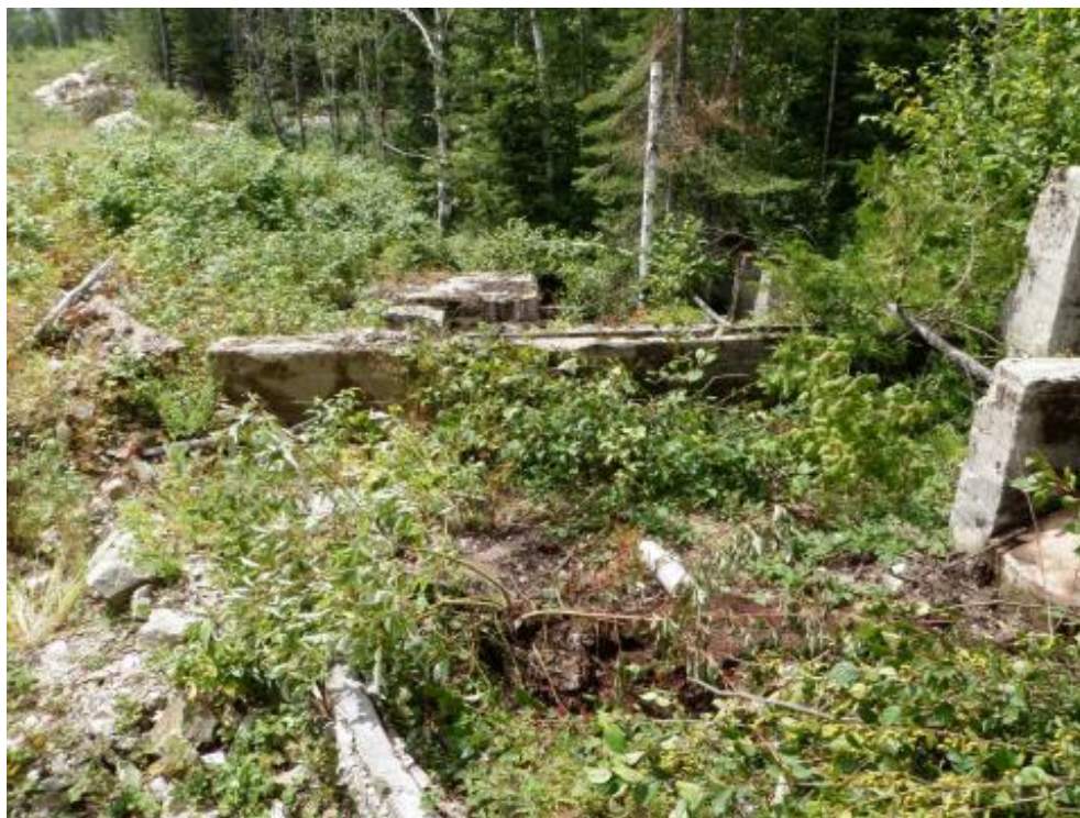
Figure 14: Northwest Corner of the Stamp Mill Foundation Looking along the South Wall of the Structure (View West)
