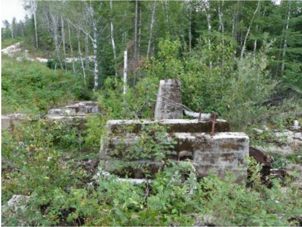
Figure 16: View of Southeast Corner of the Stamp Mill (View West)
