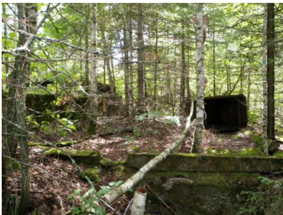
Figure 15: View of the Interior of the Structure from the Northwest Corner of the Stamp Mill Foundation (View South)
