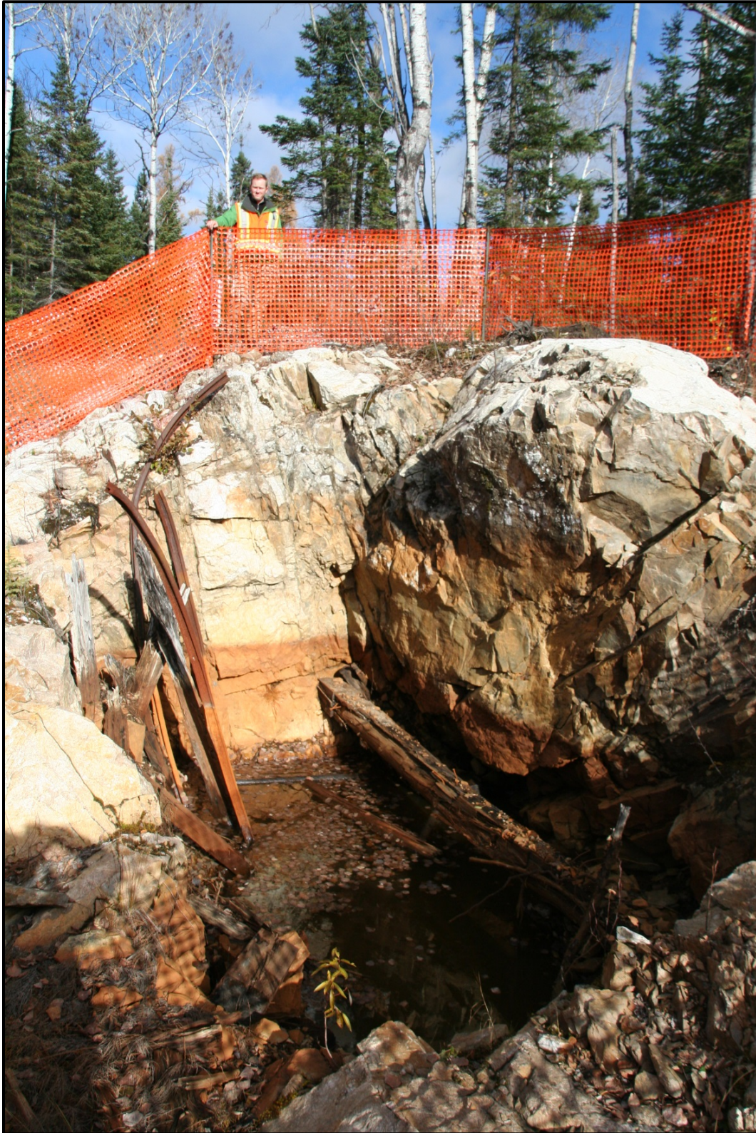
Plate S-3: Shaft One showing water in shaft, mine timber (right) and tramway rails (left)
