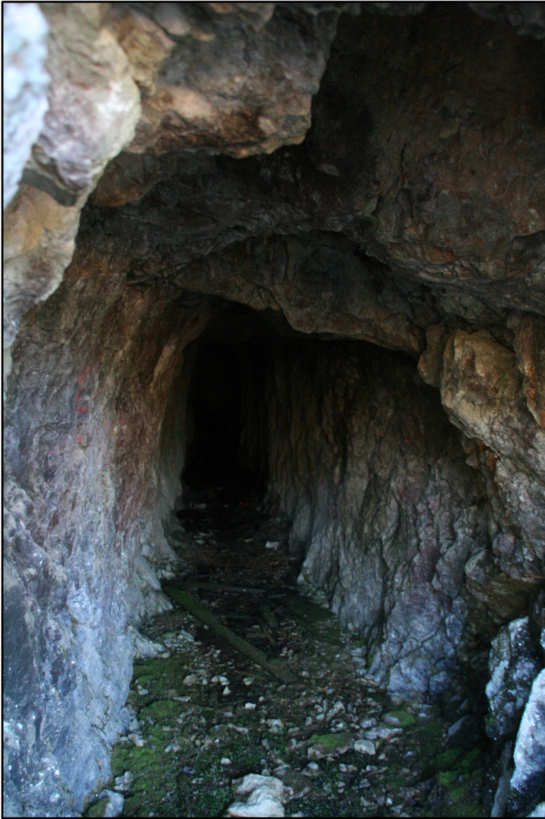
Plate H-4: Adit 2 looking from entrance; the end of tunnel is not visible
