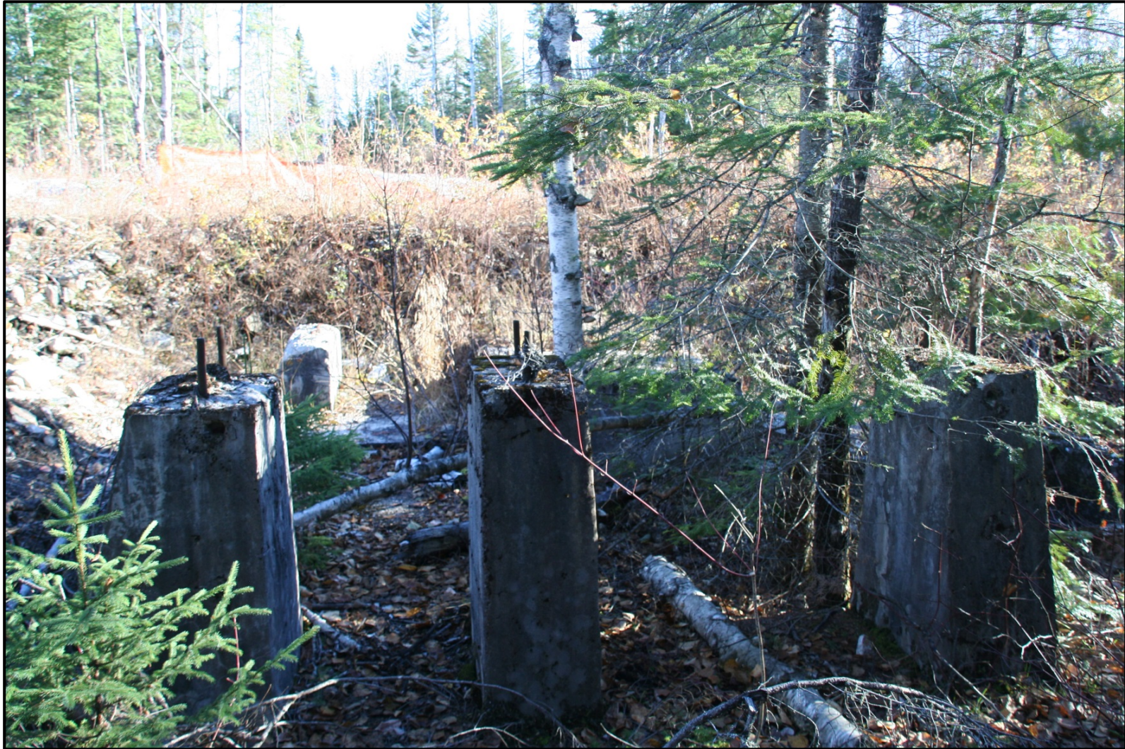
Plate S-7: Concrete footings for pillow blocks, looking towards Shaft One
