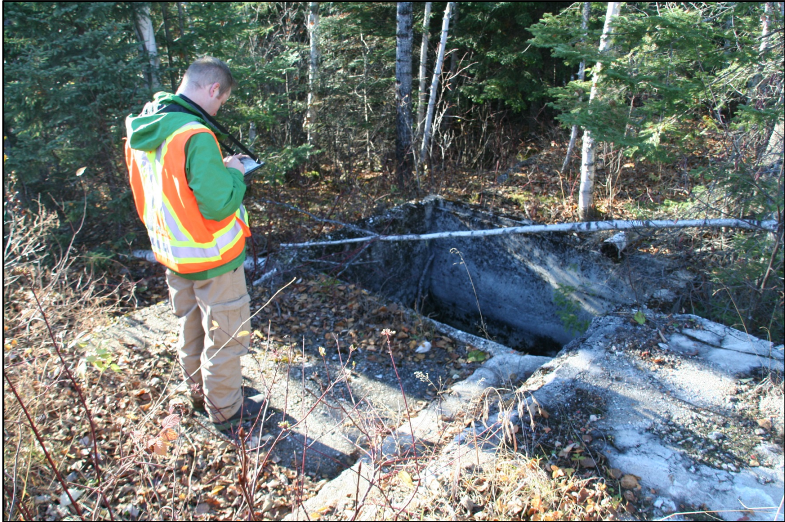
Plate S-8: Two concrete tanks on lowest level of mill foundation
