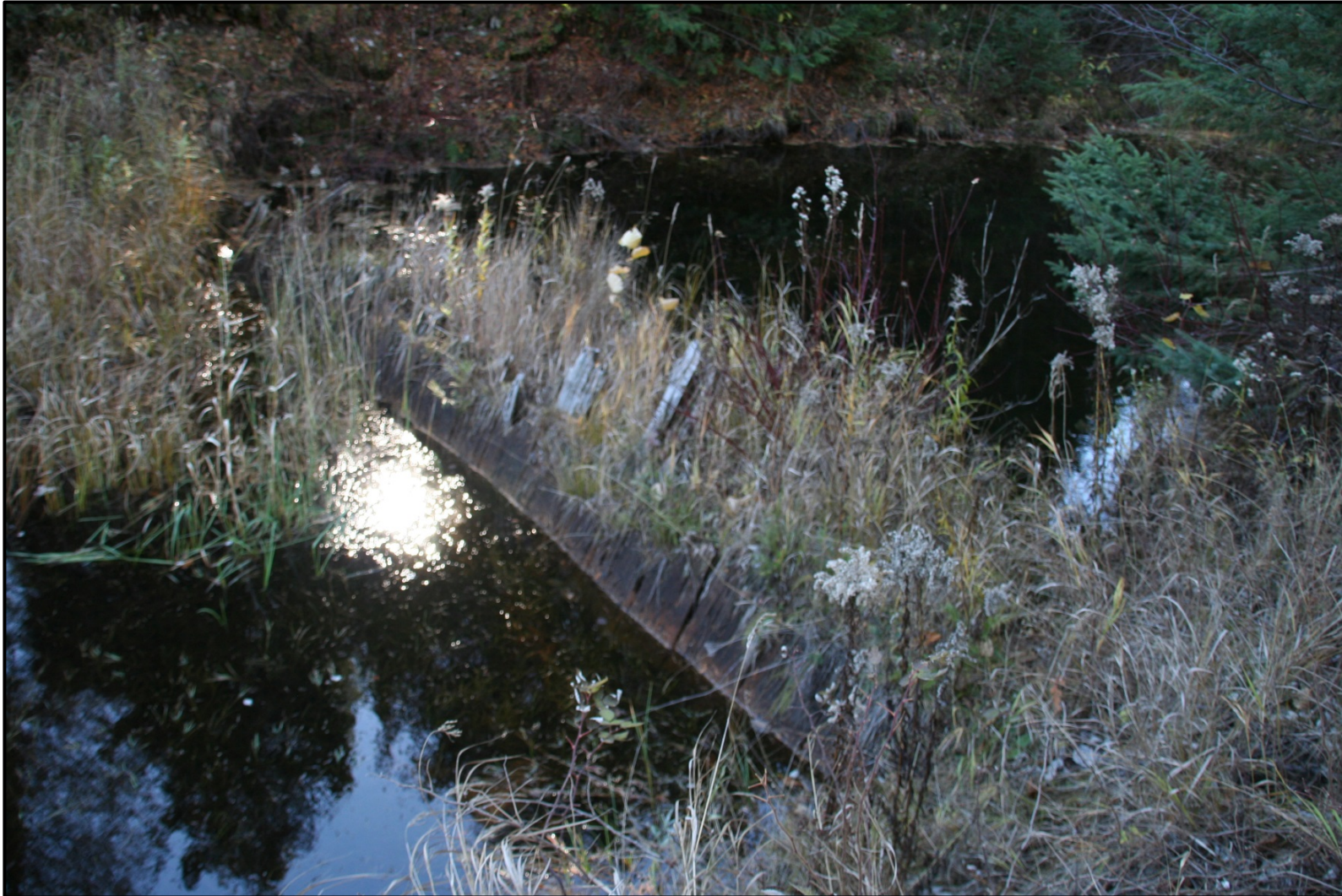
Plate H-15: Overview of dam showing timber framing on upstream side
