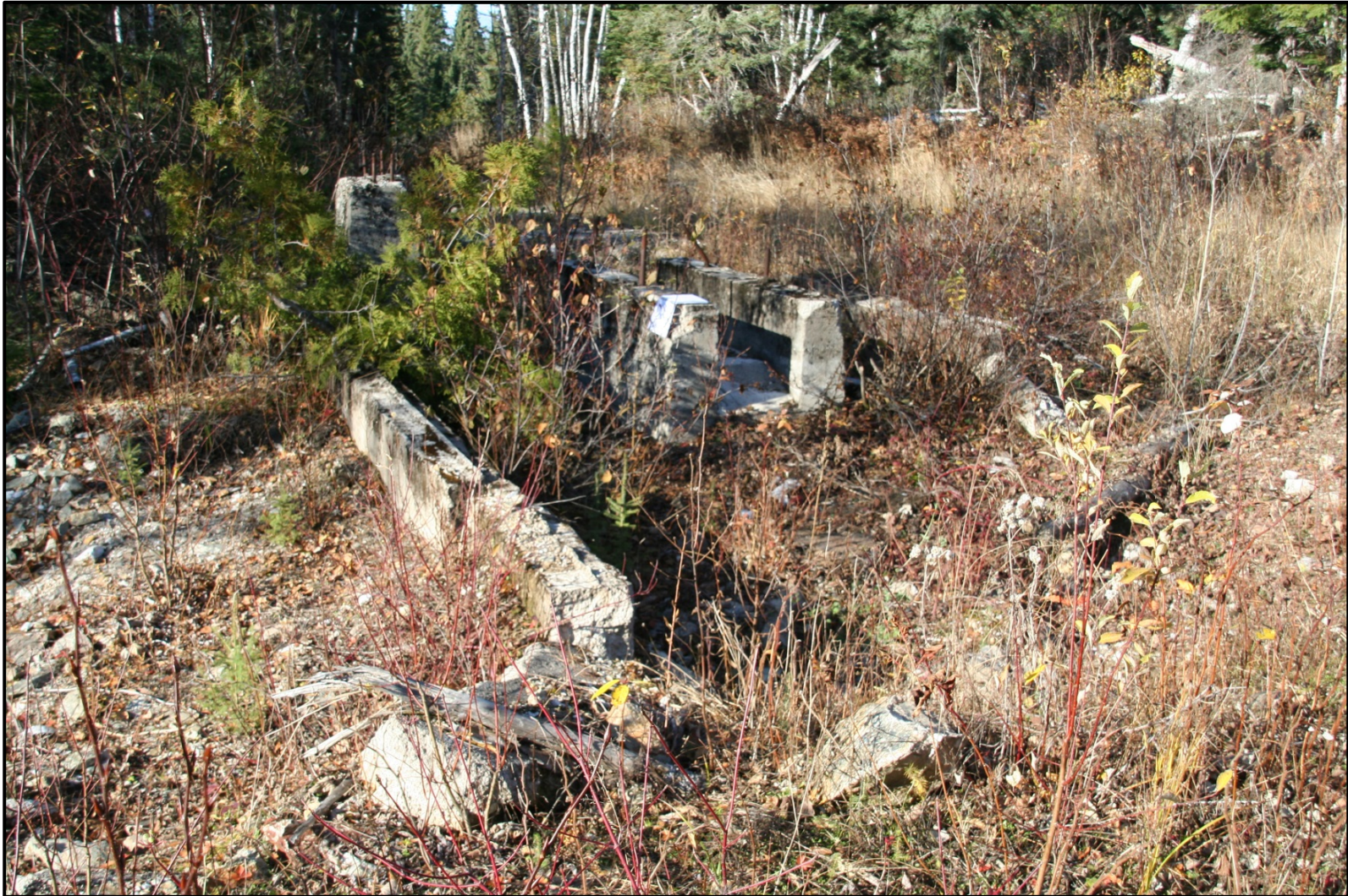
Plate S-6: Mill foundation overview looking from Shaft One
