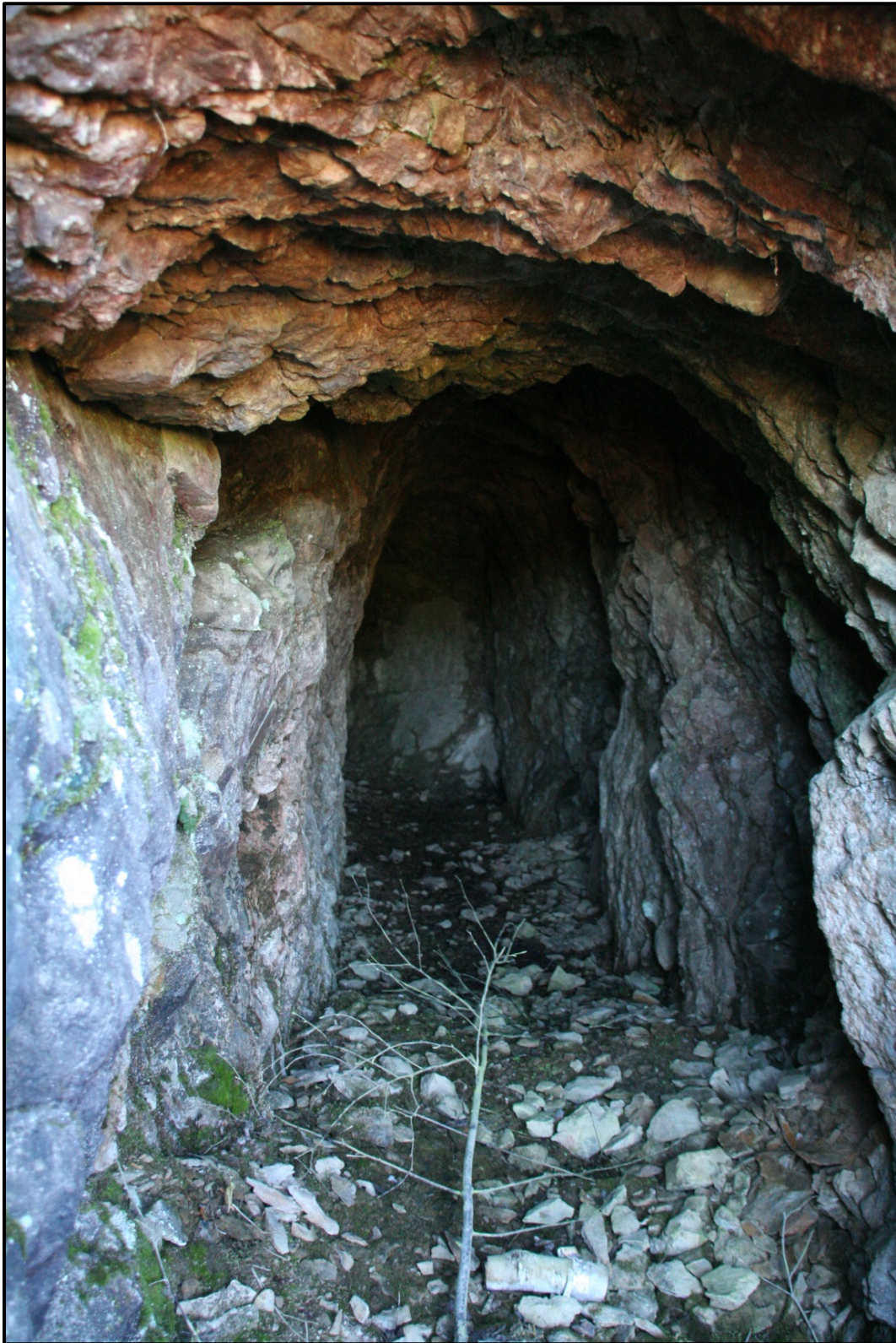
Plate H-2: Adit 1 looking from entrance with end of tunnel in rear
