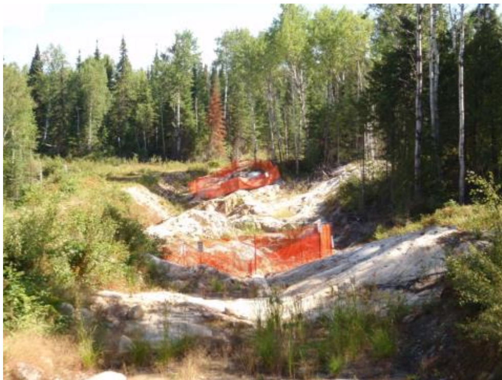
Figure 12: Main Shaft and Air Shaft from First Operation of the Mine (View Northeast)
