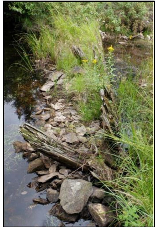
Figure 11: Close Up of Timber Crib Dam Structure, October 2011 (Source Golder Stage 1 Baseline Study and Stage 2 Archaeological Assessment 2013).
